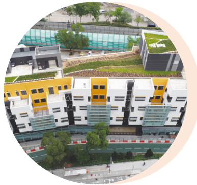
Ancillary facilities in Sheung Shui
