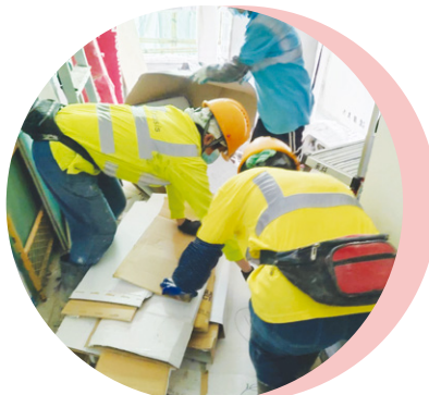
Workers helping to sort waste on site
