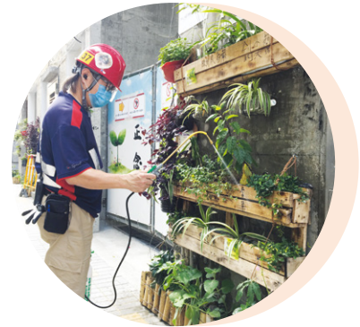
Greening the periphery of construction site
