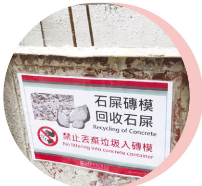
Collecting concrete for recycling
